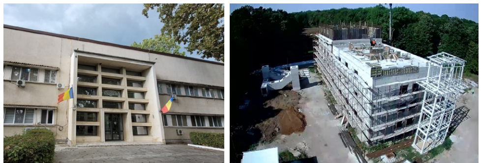
Figure 15 - The National Centre for Improving Training in Emergency Situations Management (left) visited during the peer review mission and new training facility under construction for SAR activities (right).
