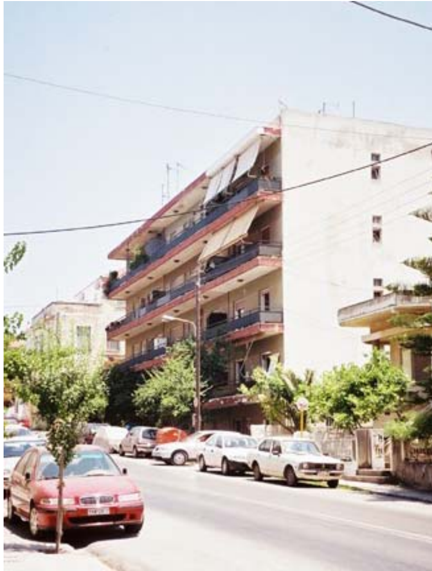
Photo 13: Building at Solomou 19 str.
