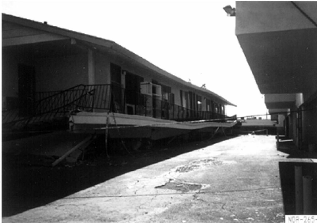
Photo 42: Collapsed 2-story wood frame apartment building (RED)
