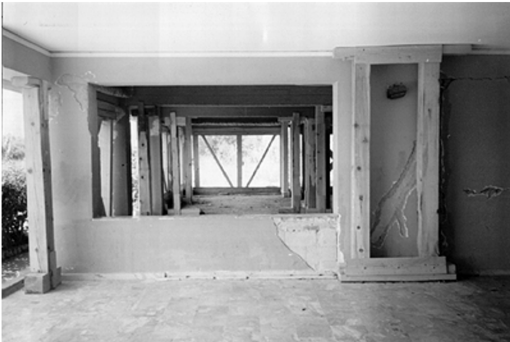
Photo 47: Emergency support of damaged open ground story of concrete building
