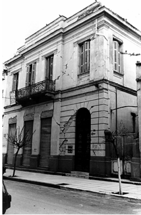
Photo 29: Moderate to heavy damage (YELLOW)
