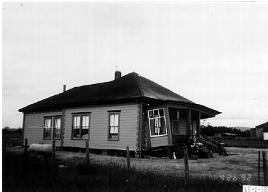
Photo 41: Single story wood frame house slipped off its foundation (RED)
