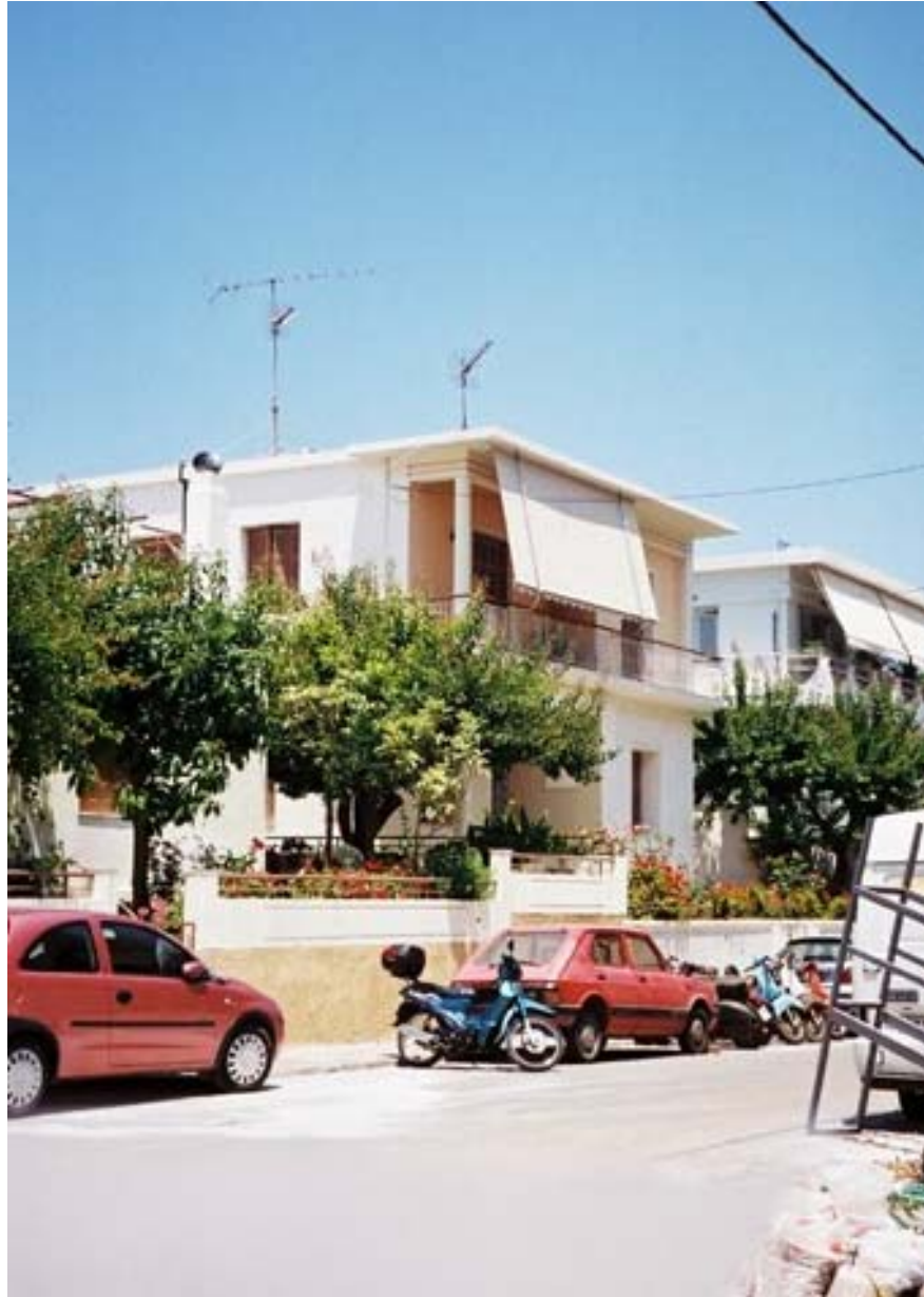
Photo 7: Building at Kriaradon 8, str.
