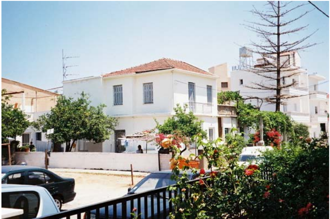
Photo 8 : Building at Mandaka 10 str.
