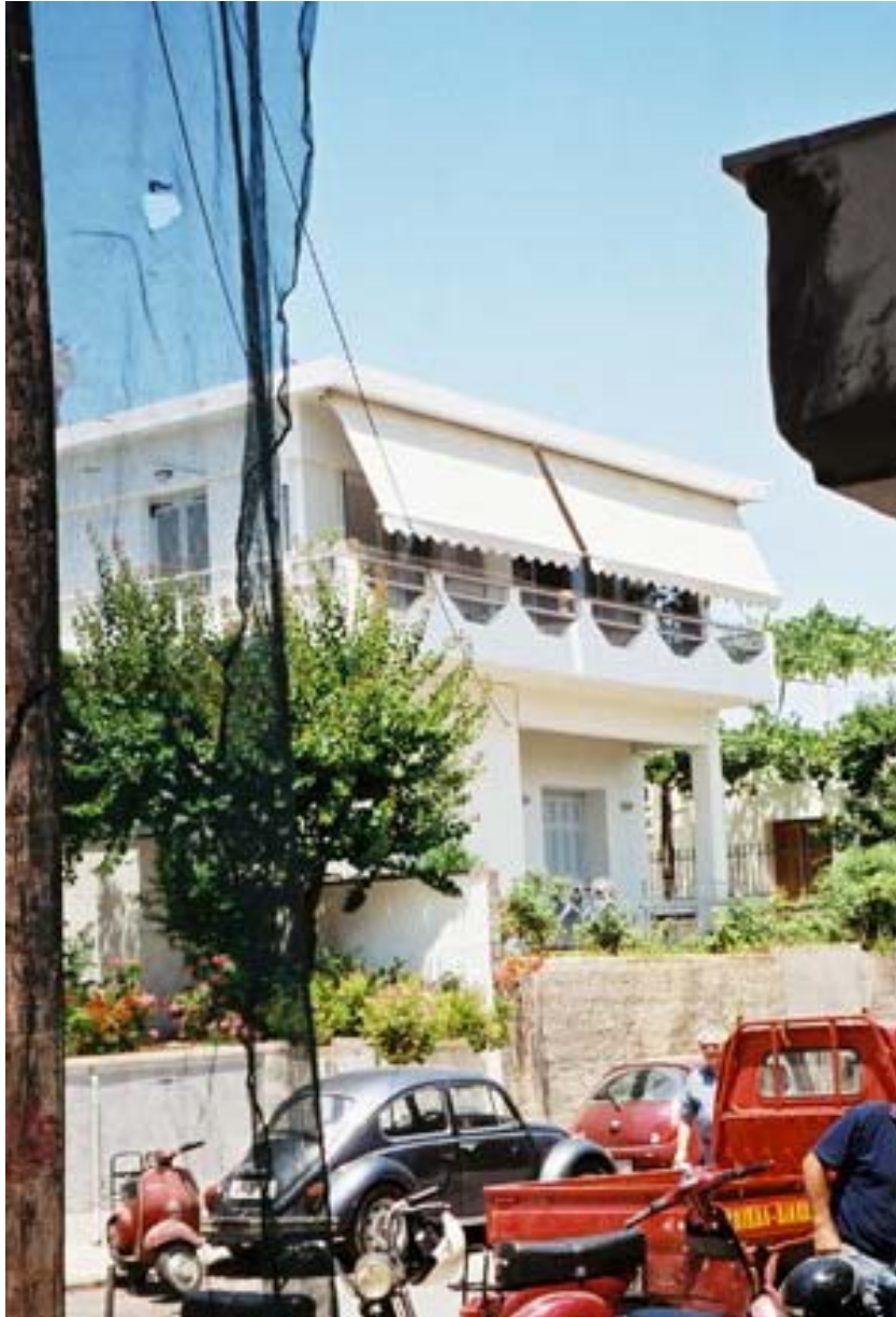
Photo 6: Building at Kriaradon 6 str.
