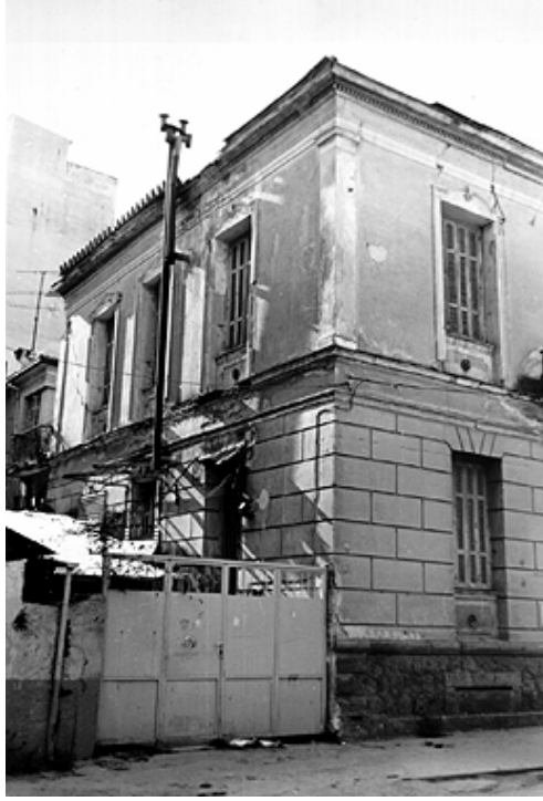
Photo 27: Slightly damaged (GREEN)
