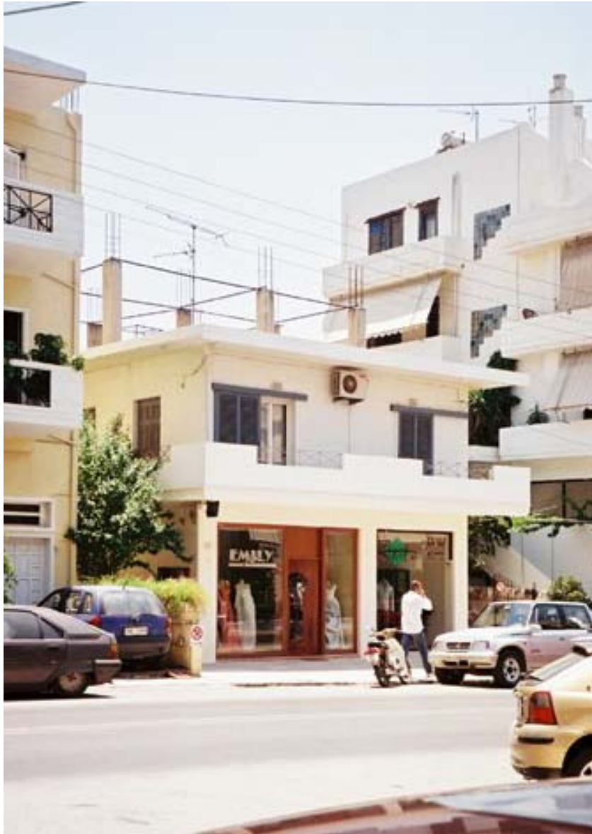
Photo 15: Building at Solomou 27 str.
