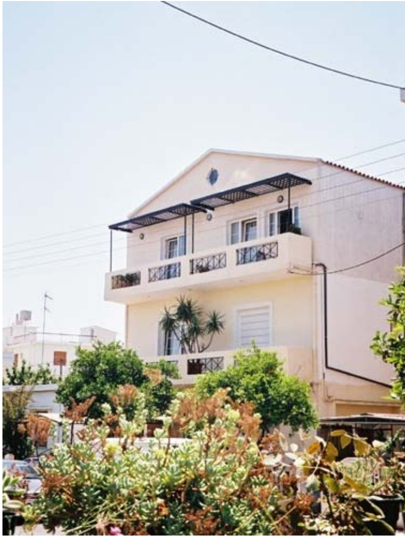
Photo 12: Building at Skoula 21 str.
