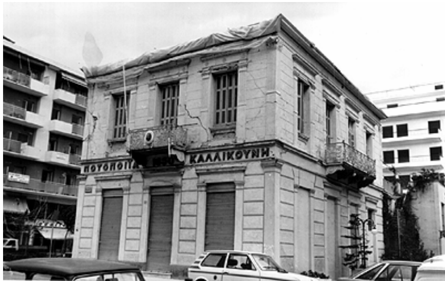
Photo 28: Slightly damaged (GREEN)
