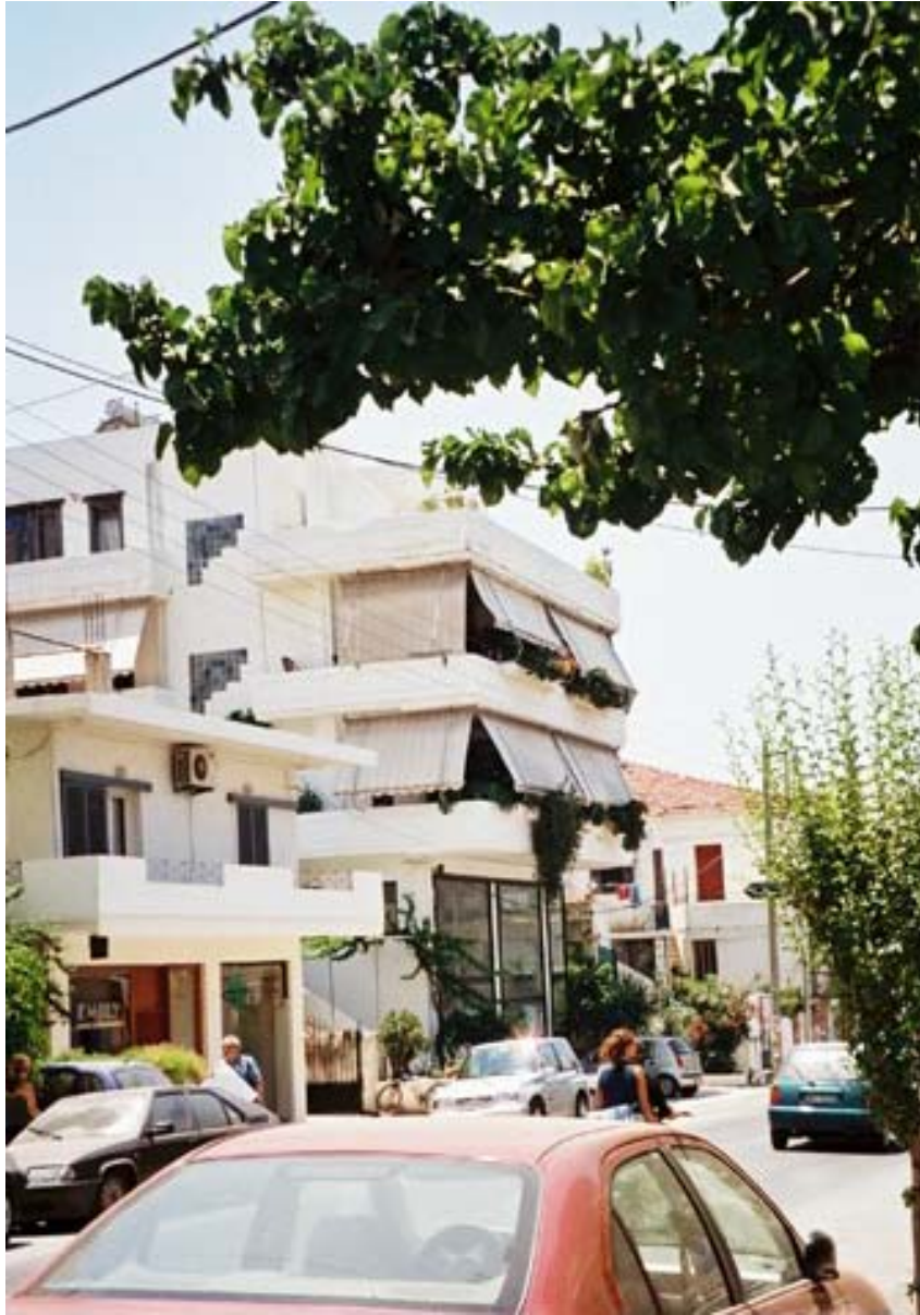
Photo 16: Building at Solomou 29 str.
