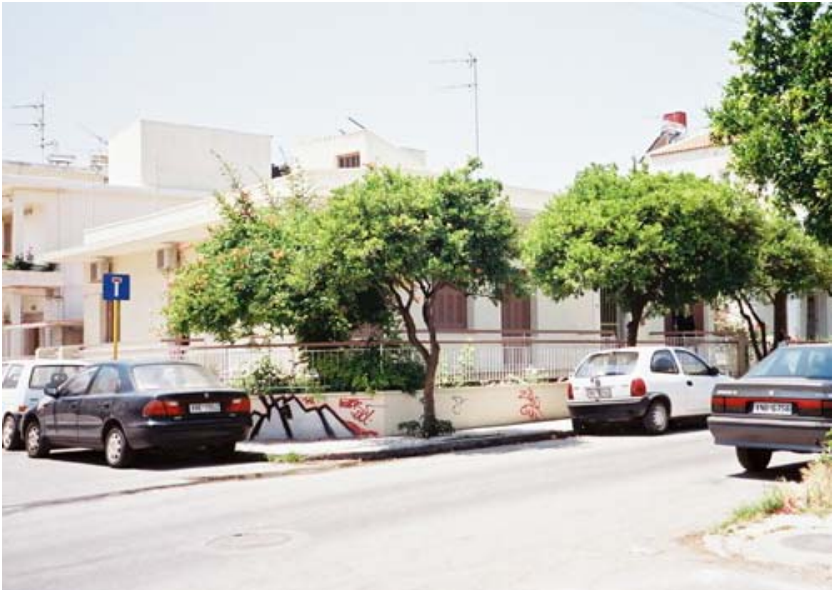
Photo 10 : Building at Skoula 17 str.
