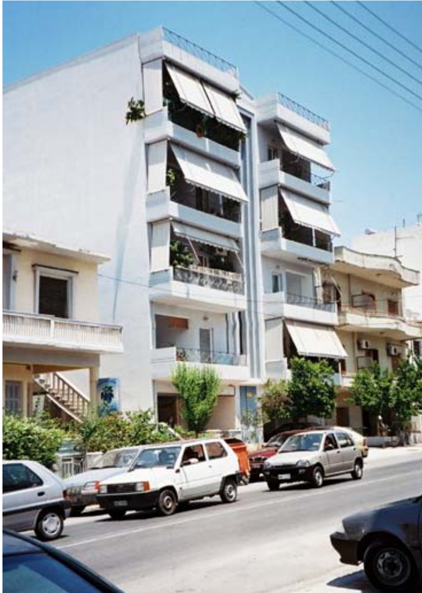
Photo 5: Building at Solomou 22 str.
