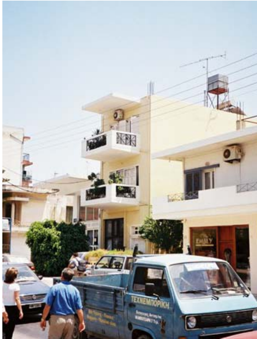
Photo 14: Building at Solomou 25 str.
