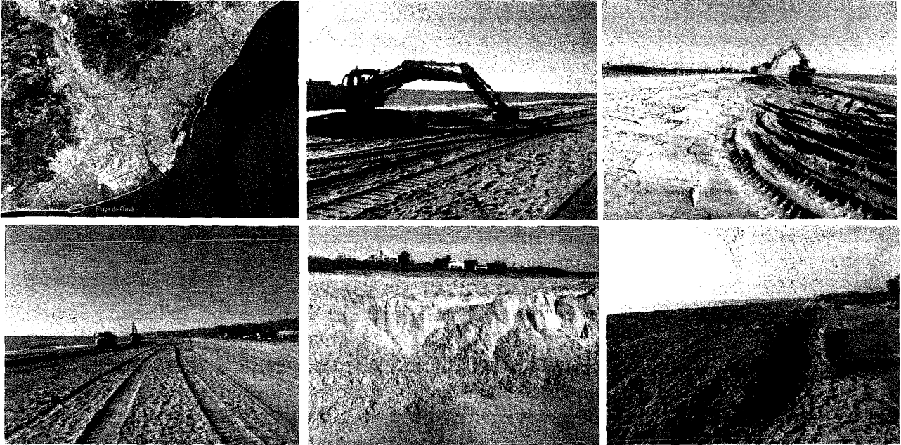
Figure 9. QDM construction process at Gava during December 2015
