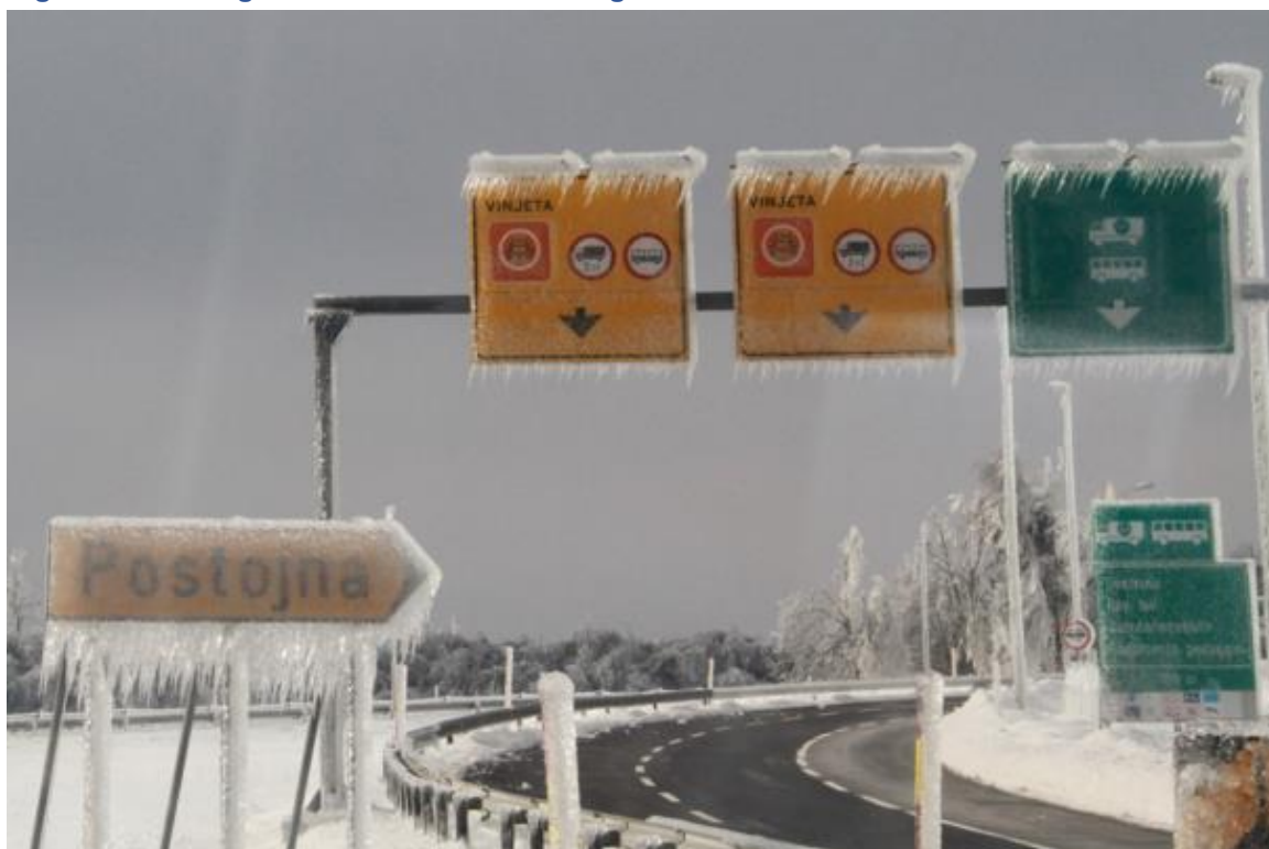
Figure 19: Damage at installation of road signs
