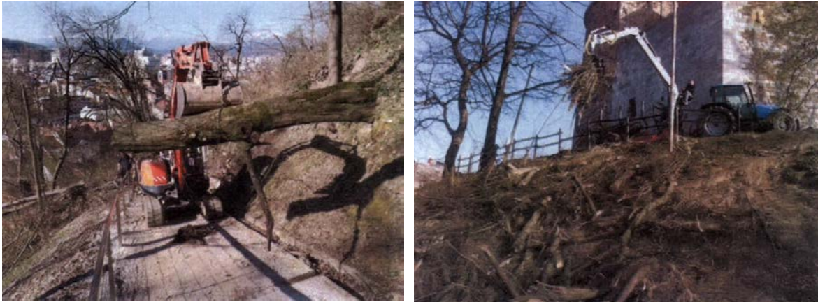
Figure 20: The temporary safety nets
