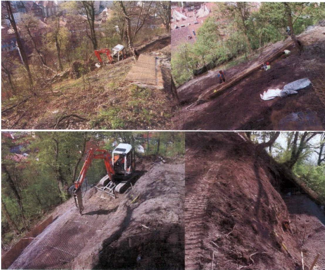
Figure 21: The reinforced slope
