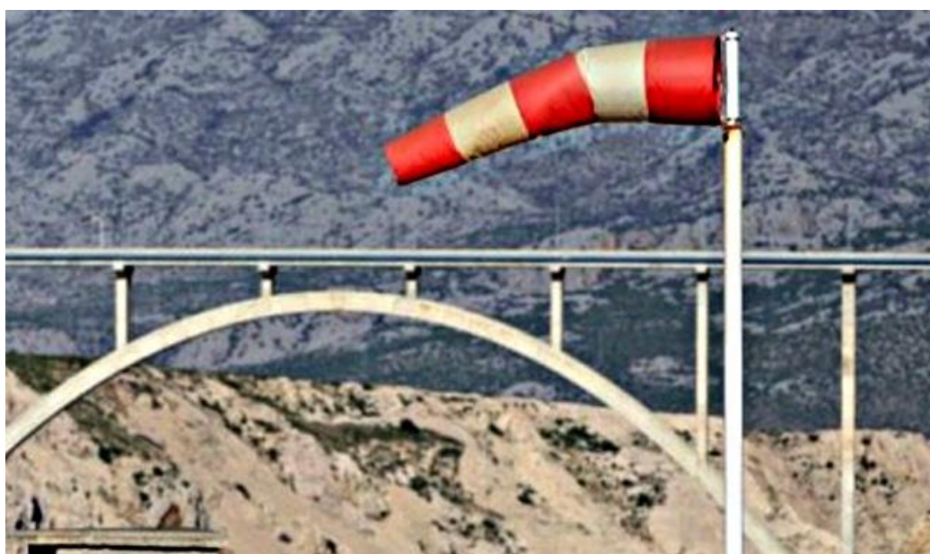
Figure 10: High wind over the bridge
