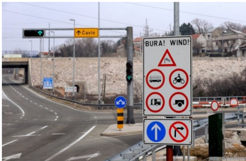
Figure 9: Closing the part of the road due to the high wind conditions
