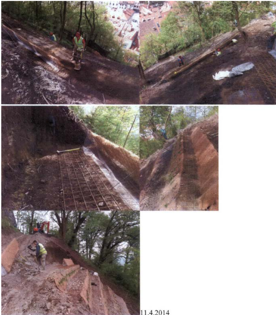
Figure 23: The reinforcing of slope in different time phases
