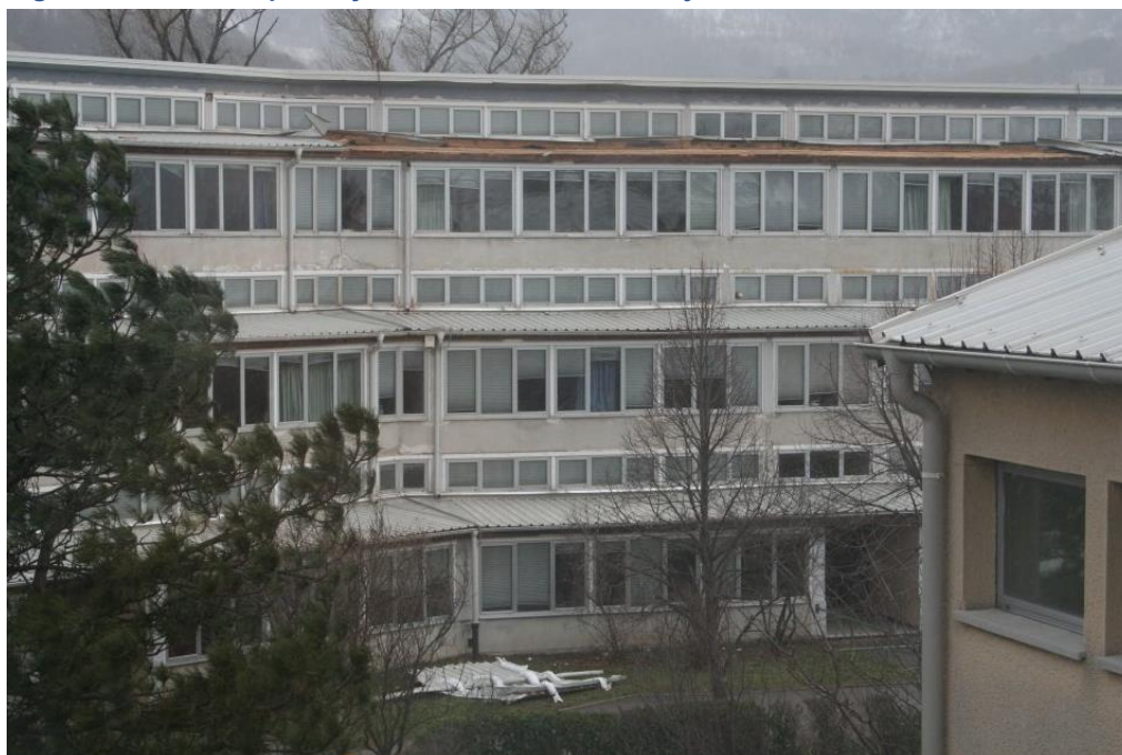
Figure 29: Unroofed primary school Danilo Lokar in Ajdovščina
