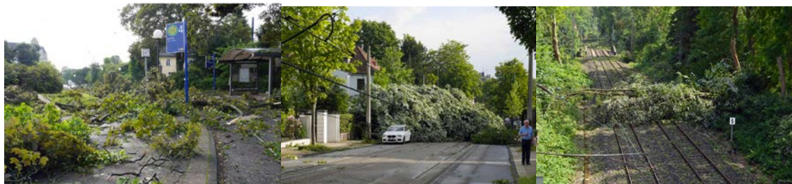
Figure 10: Damages to roads, rail network and train stations
