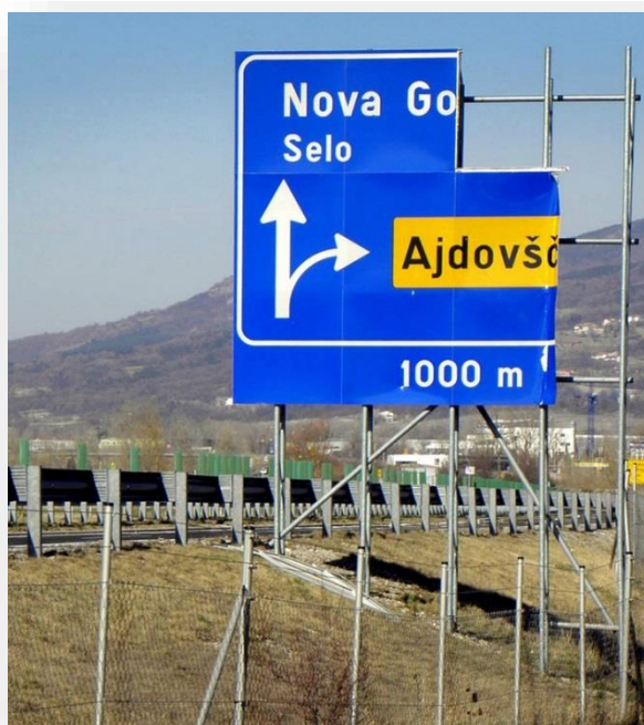
Figure 5: Damaged traffic sign on the regional motorway as a consequence of bora wind 24
