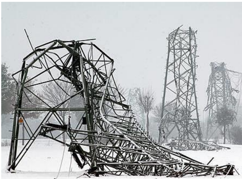
Figure 32: Collapse of electricity pylons during the Münsterländer Snow Chaos
