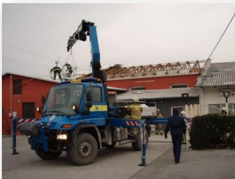
Figure 4: Roof restoration after Bora event 20
