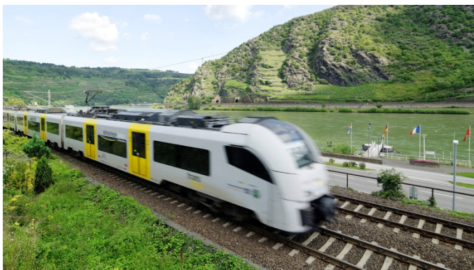
Figure 38: Rail tracks in highly exposed winter storm area
