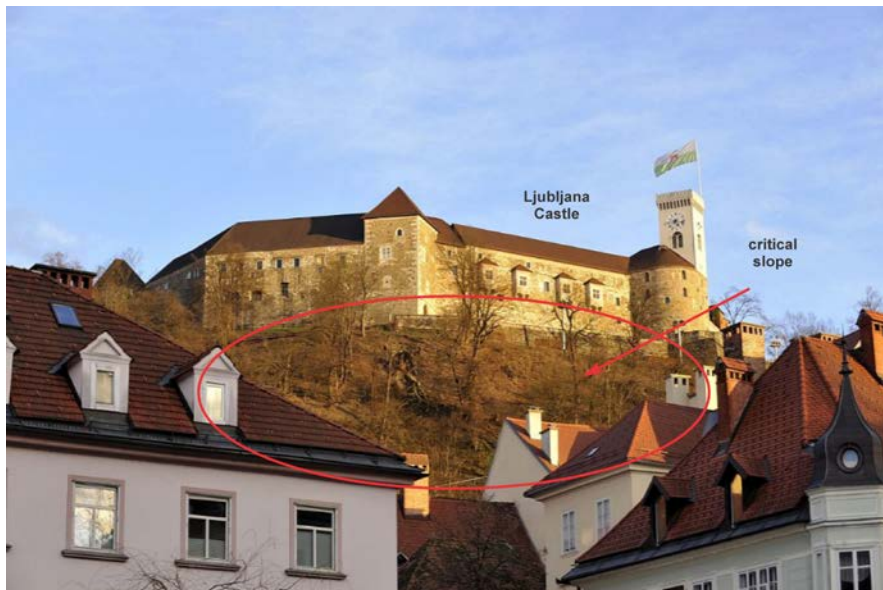
Figure 17: The critical slope below Ljubljana castle
